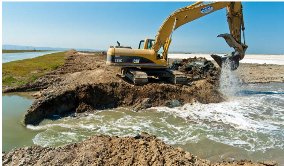
Levee being breached and tidal flows restored at Eden Landing in Hayward. Photo by SBSPRP.
