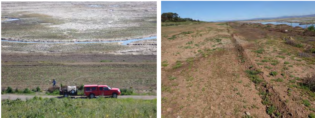
Figure 3.2-2. The newly constructed ecotone levee (Ravenswood, South Bay Salt Pond Restoration Project) at the south side of Bedwell Park is in the first growing season of revegetation after planting and seeding by Save The Bay, March 11, 2022. During this period of high vulnerability to wind-wave erosion while vegetative stabilization is incomplete, the levee is not exposed to tides and wind-waves, prior to tidal restoration. This sequence contrasts significantly with the proposed West Bay ecotone levee plans.
