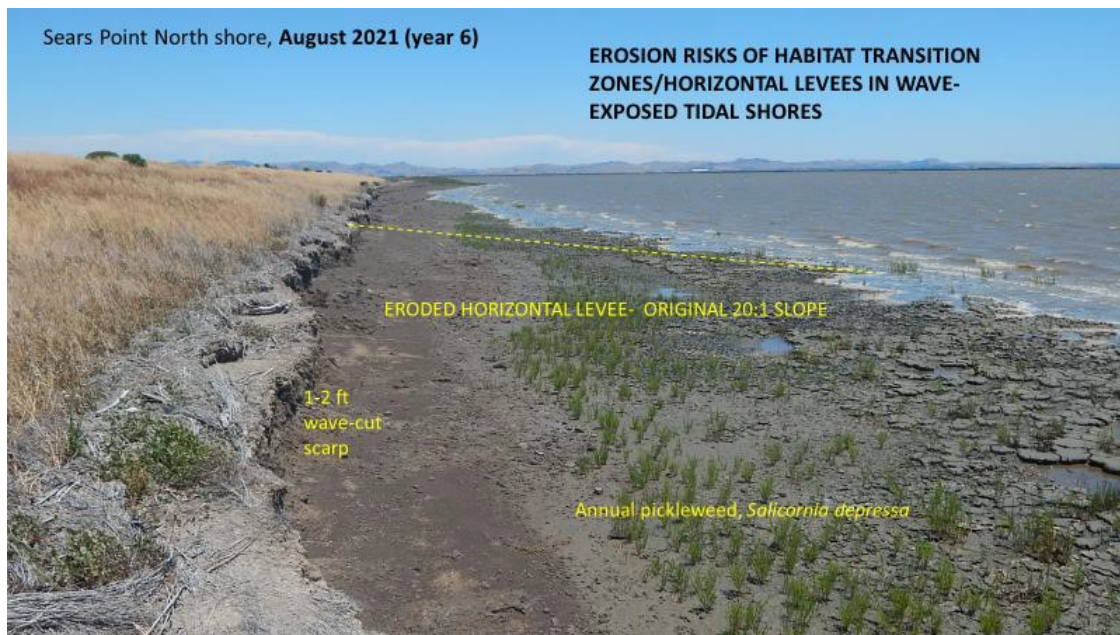
Figure 3.2-1. Sears Point Wetland Restoration Project ecotone levee wind-wave erosion 3-6 years after construction. San Pablo Bay National Wildlife Refuge. Ecotone slope erosion was severe, leaving a wave-cut bench with the Mean High Water line close to the eroded scarp by 2021.
