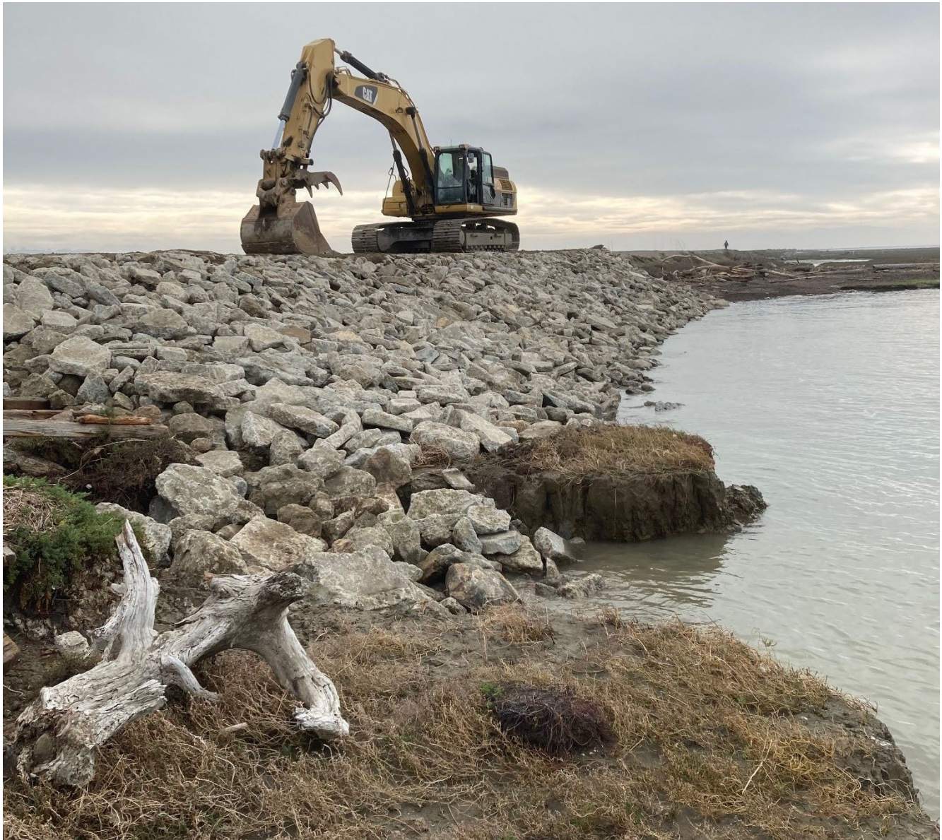
Figure 206. Riprap Placed on Outboard Side of Berm
